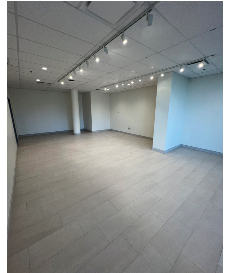
CURRENT UNFINISHED SPACE FOR THE FRICTIONLESS STORE-LAB. RENOVATIONS ARE ONGOING.
